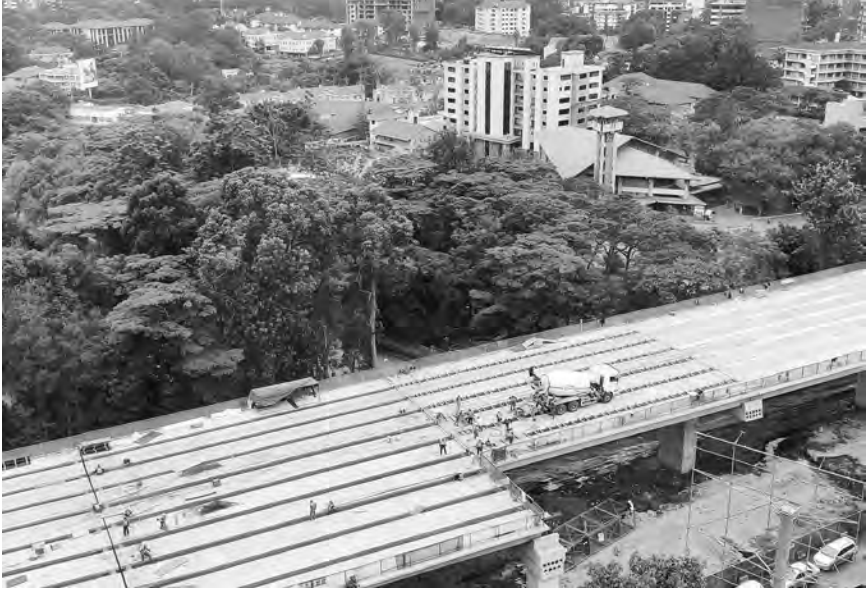
FIGURE 10. The Nairobi expressway under construction. Photo by author.
