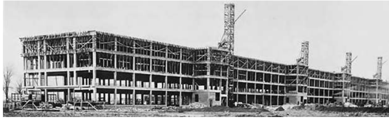
Fig. 7.1. Ford Motor Company Plant, Highland Park, Detroit. Prime Officine. Costruzione 1909-1910, www.generi-carchitecture.org.
