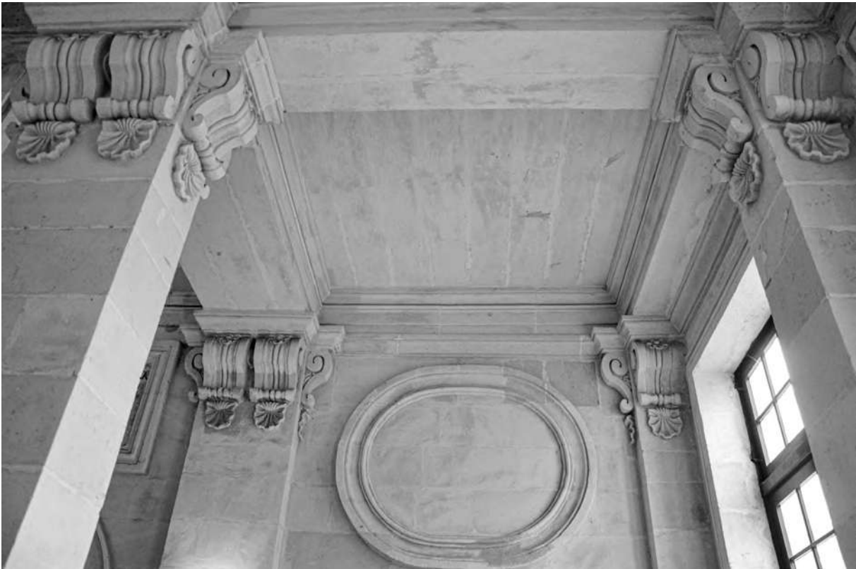
Figg. 13-14. Constructive details with the lintels made of monolithic stone blocks [photo by Armando Antista, 2022].
