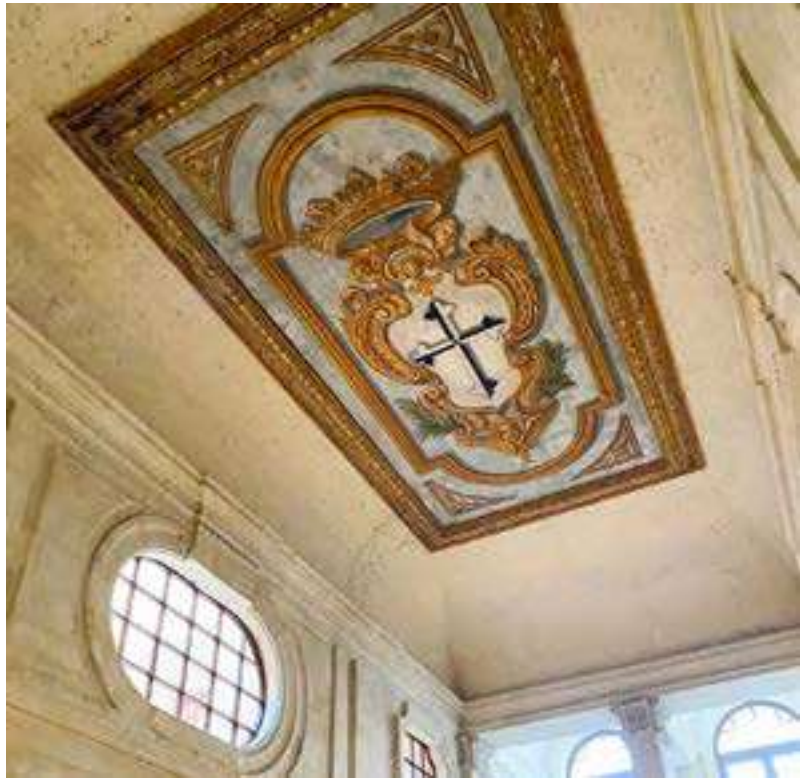
Fig. 15. The lowered pavilion-headed vault with the central decoration [photo by the author, 2022].
