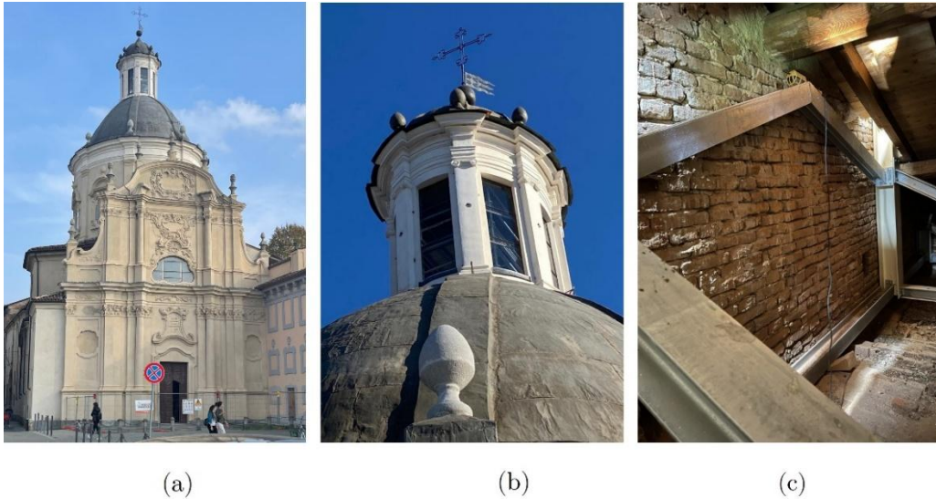
Figure 1.3. Church of Santa Caterina: (a) global view, (b) intervention on the lantern, and (c) intervention of the façade.
