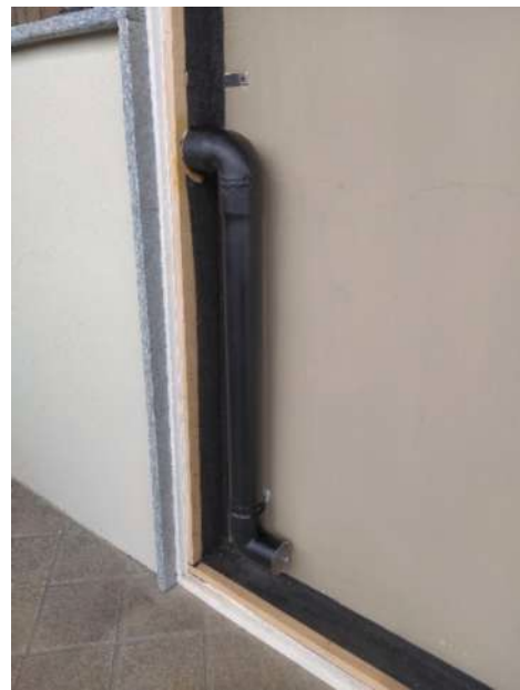
Fig. 4. Inlet pipe installed in Wall A and Wall C.
