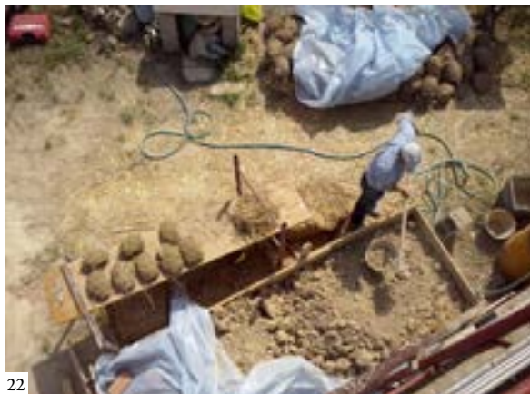
Figure 23: Laying of massoni by workshop participants: they can be thrown with force, to allow the release of excess water, or laid on beds of dry straw and pressed to adhere and penetrate each pore (CEDTerra)
