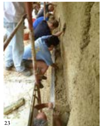
Figure 23: Laying of massoni by workshop participants: they can be thrown with force, to allow the release of excess water, or laid on beds of dry straw and pressed to adhere and penetrate each pore (CEDTerra)
