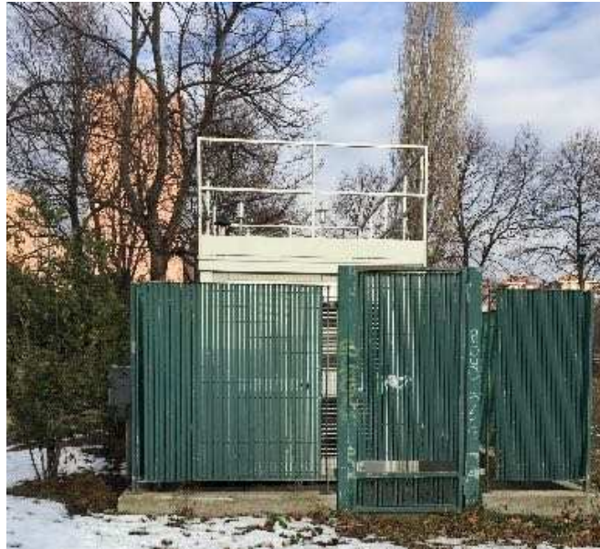
Fig. 3.1 High-precision monitoring station - Rubino station in Turin- Italy
