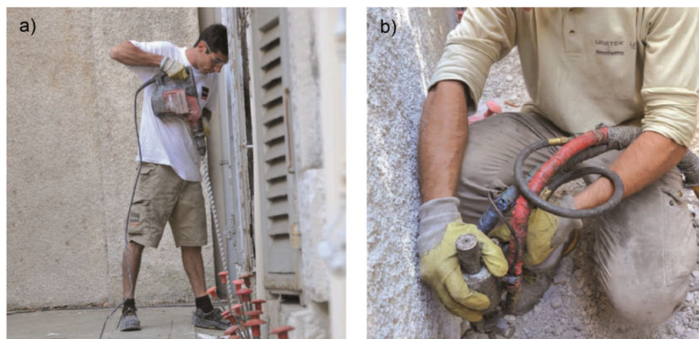
Figure 1. Example of operations: a) Drilling of the borehole; b) Equipment for the injection of the expanding polyurethane resin.
