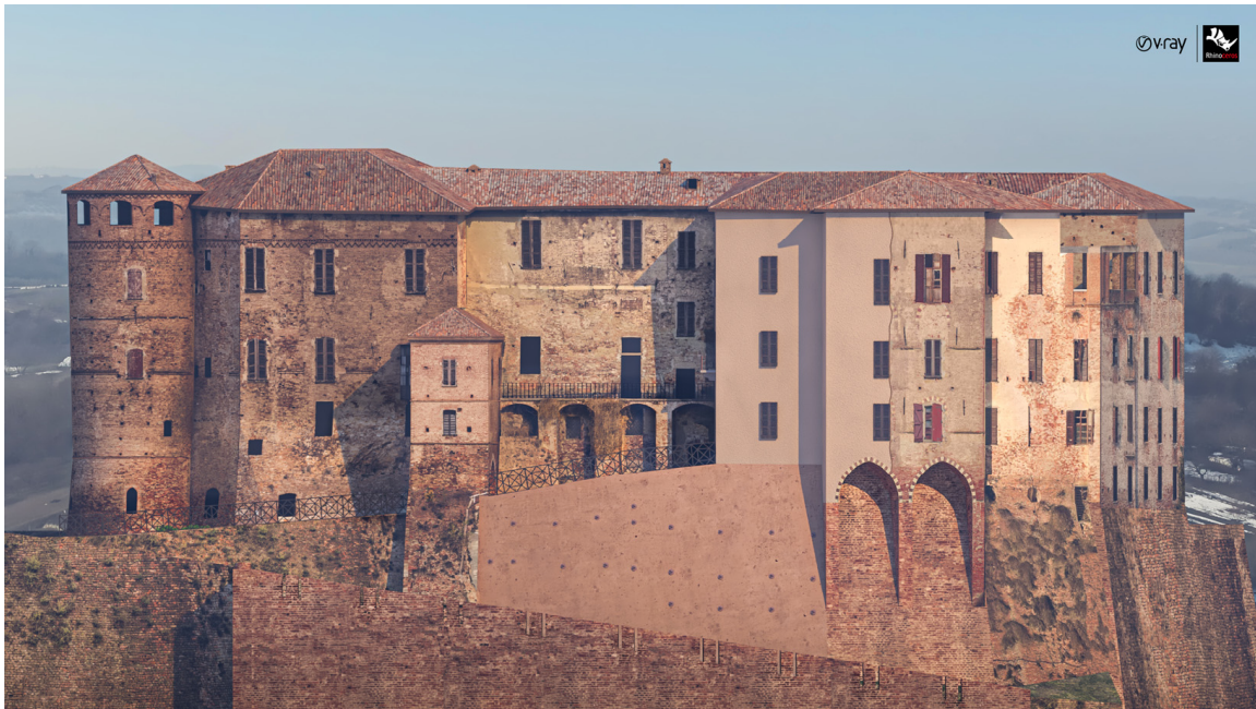
Figure 26. The 3D-rendered model proposed for reconstructing the collapsed area: modelled with Rhinoceros and V-Ray. South front of the castle.
