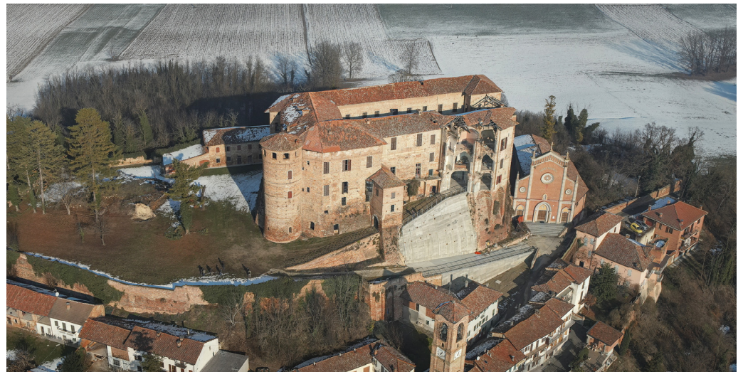
Figure 3. Aerial image of the Frinco Castle from the south side, from which the collapsed area is visible.
