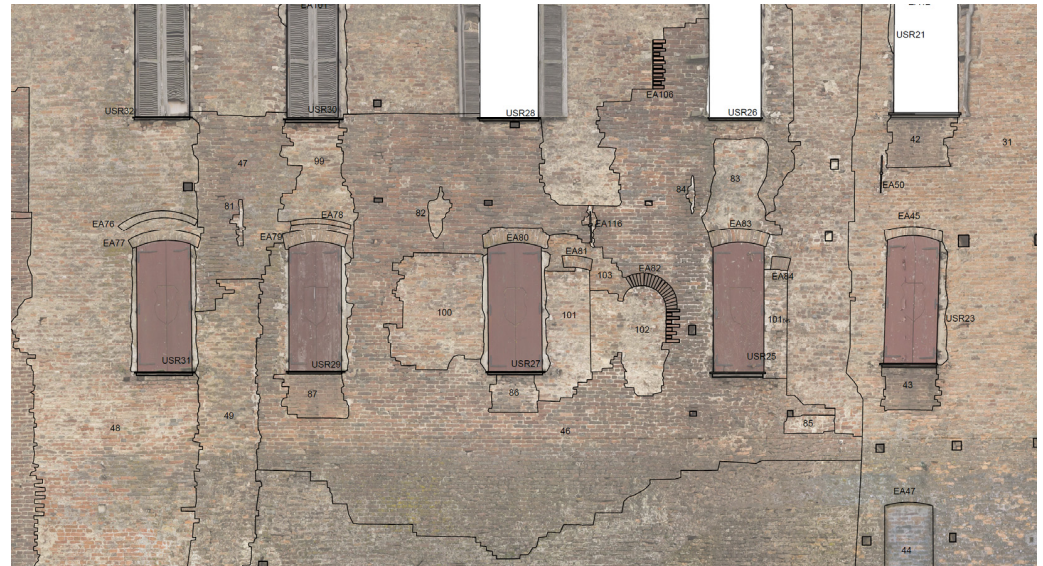
Figure 7. Stratigraphic units' detection in the castle's north front (small portion). Different masonries, openings, and other architectural and structural elements can be noticed.
