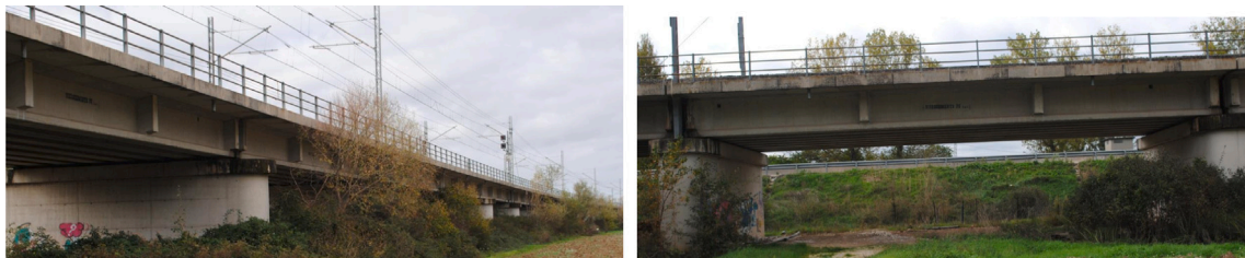
Fig. 10. Views of the viaduct and of a sample span.
