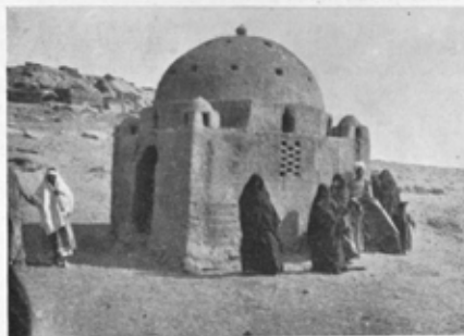
Mud-brick Tomb, near El Kab, Upper Egypt.
