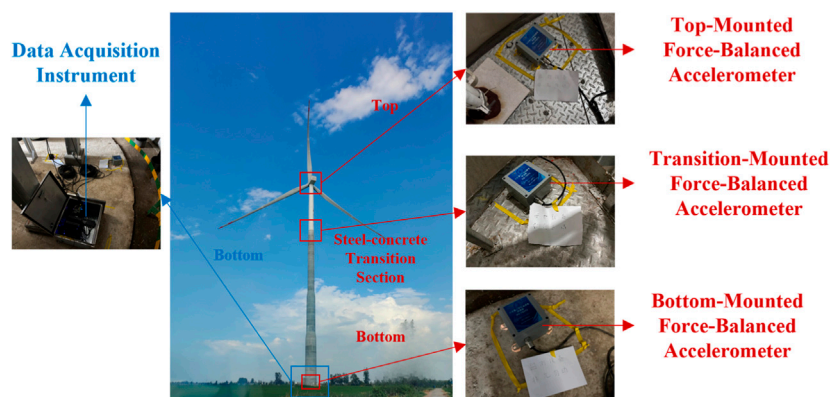
FIGURE 1 Overall architecture of wind turbine hybrid tower monitoring system.
