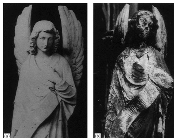
Figure 6. Influence of biodeterioration processes occurred on an angel statue at the "Peters"-Portal on the Cathedral of Cologne (Germany): a) original object in 1880 photograph; b) the respective weathered statue in 1993. Reproduced with permission. [23] Copyright 2000, Elsevier.
