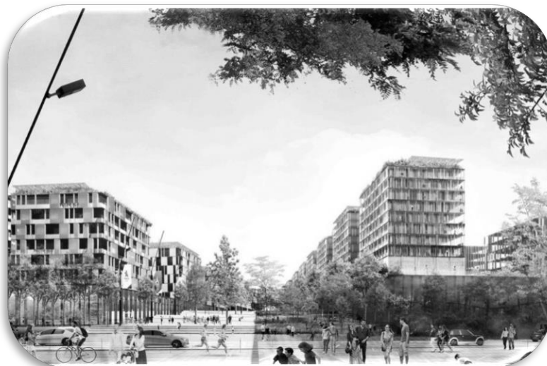
Figure 89 Paris 2024 Olympic Village Project (Source: COJO,2024)
