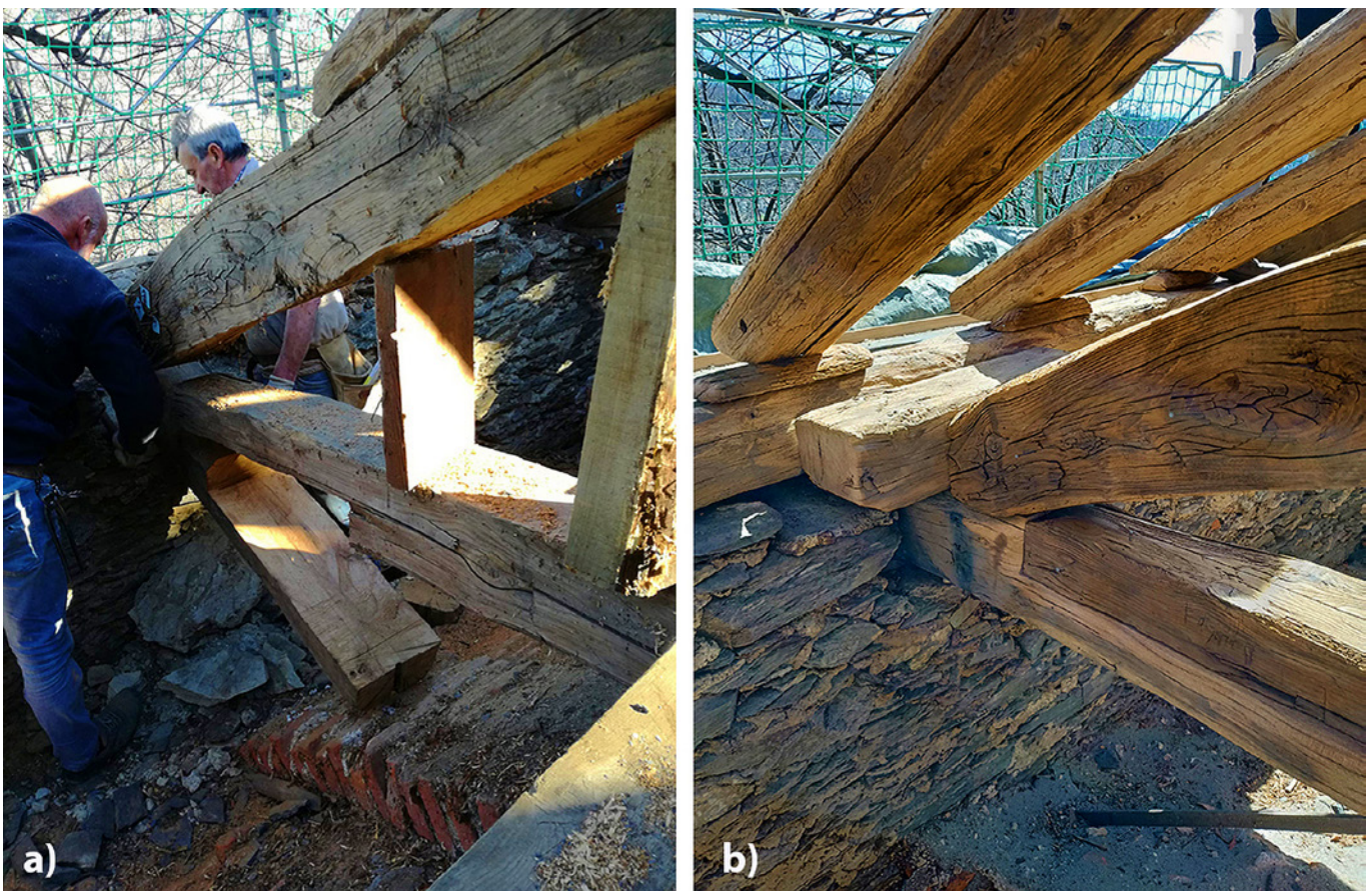
Fig. 9. (a) Positioning of the timber prosthesis; (b) the timber-timber prosthesis performed.
