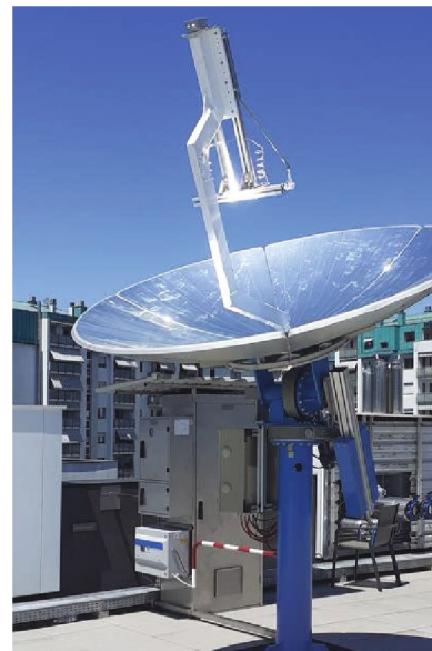
FIGURE 2: Solar parabolic dish prototype installed at the Energy Center rooftop.
