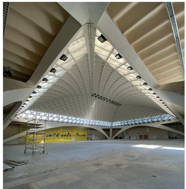
Figure 2 | View of the interior of Hall C, where it is also possible to appreciate the detail of the inclination of the arches supporting the vault and perimeter slabs.
