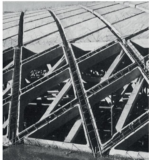
**Figure 3** | Detail of the site during the construction phase of the ribbed pavilion vault. In the image it is possible to see the hollows for the casting of the ribs. Università di Firenze, Biblioteca di Scienze Tecnologiche (BST) - Archivi di Architettura, Fondo Pier Luigi Nervi (024-2783).
