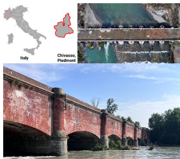
Figure 1. The Cavour Canal water bridge over the Dora Baltea River (Saluggia, Italy), a 19th-century masonry hydraulic structure characterized by a multi-arch configuration and a continuous water conveyance system.
