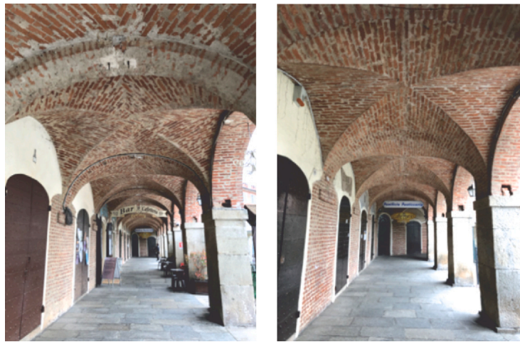
Fig. 2. View of two different 18th century vaults of the portico, with radial masonry pattern (right) and diagonal pattern (left).
