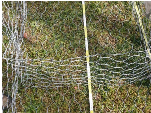
Figure 134 : Fixing the bracing meshes
