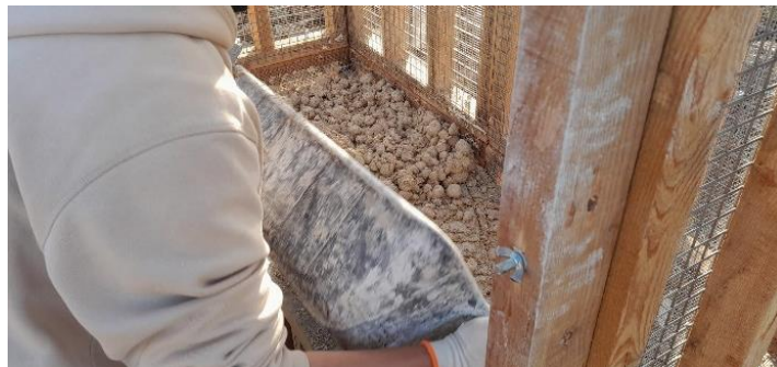
Figure 74 : Filling the formwork with hemp-lime
