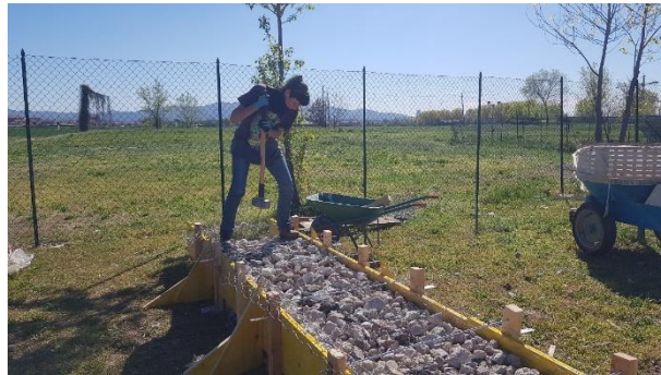
Figure 141 : Smashing the rubble for compaction
