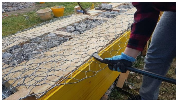
Figure 144 : Closing the gabion edge
