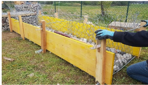
Figure 137 : Preparing the grid in the formwork
