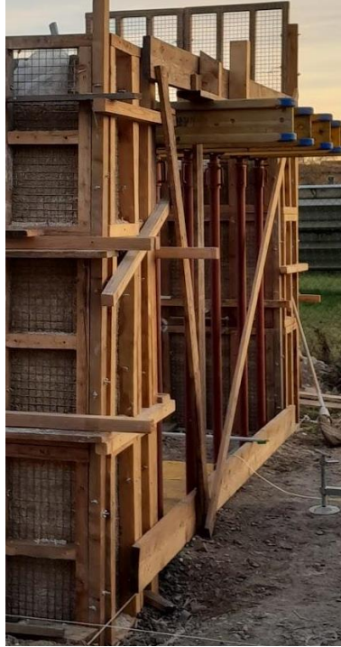
Figure 73 : Bracing between the piers
