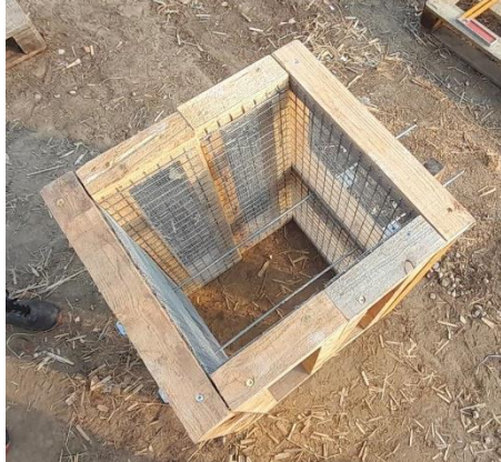
Figure 62 : Tested formwork waiting to be filled
