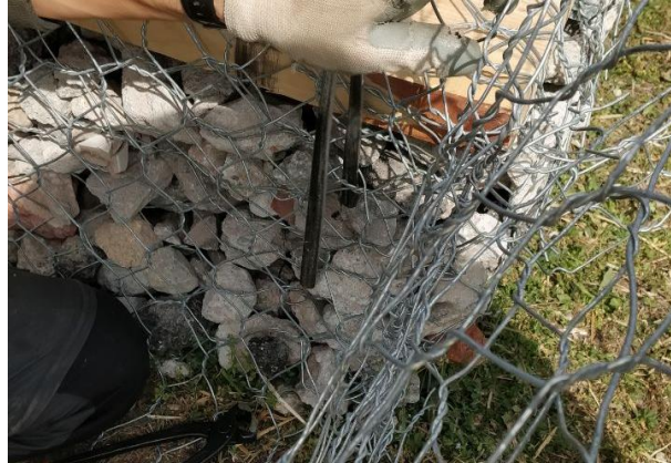
Figure 135 : Attaching gabions together
