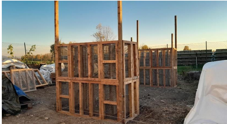
Figure 71 : Pouring in the piers formworks
