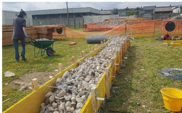
Figure 140 : Filling the gabions
