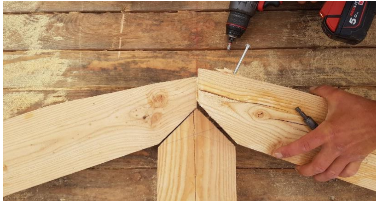
Figure 58 : Junction of wooden parts
