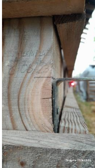
Figure 145 : Laser measurements of settlement
