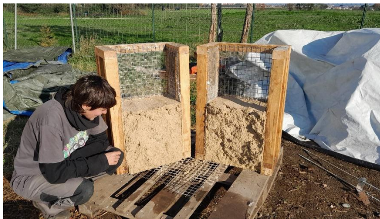
Figure 64 : Opening the formworks
