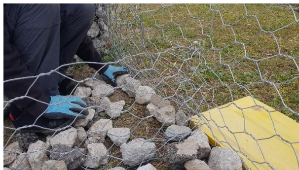
Figure 136 : Positioning the first stones by hand
