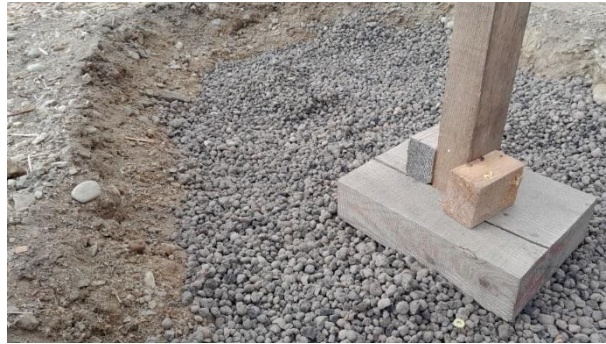
Figure 69 : Expanded clay compaction
