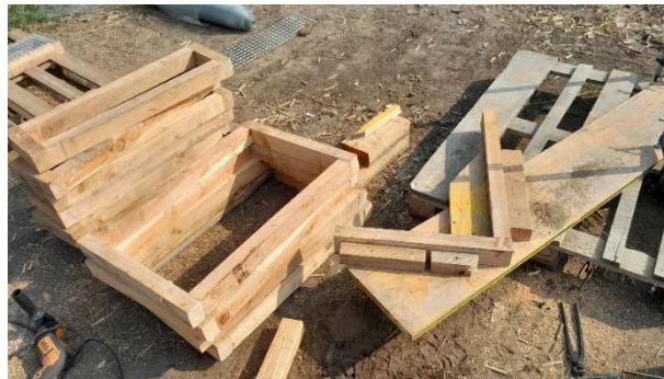
Figure 57 : Building frames of the formworks
