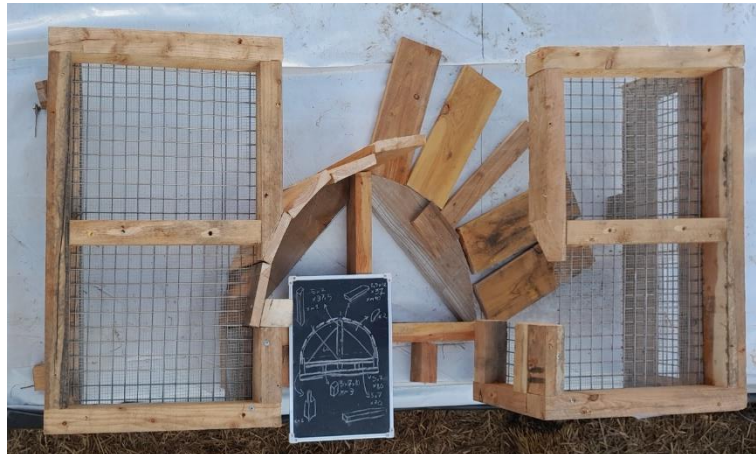
Figure 56 : Formwork of the transversal little arch
