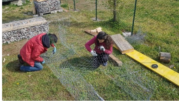
Figure 133 : Fixing the fence by hand
