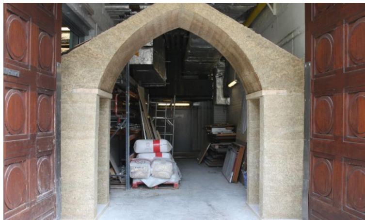
Figure 45 : Vault made in hemp-lime at Cardiff University (2009)
