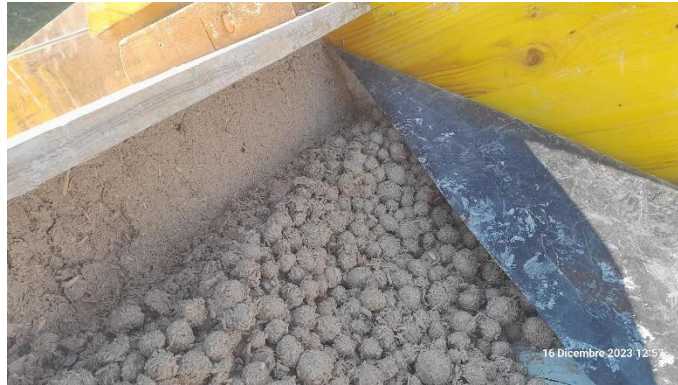
Figure 83 : Mix during compaction
