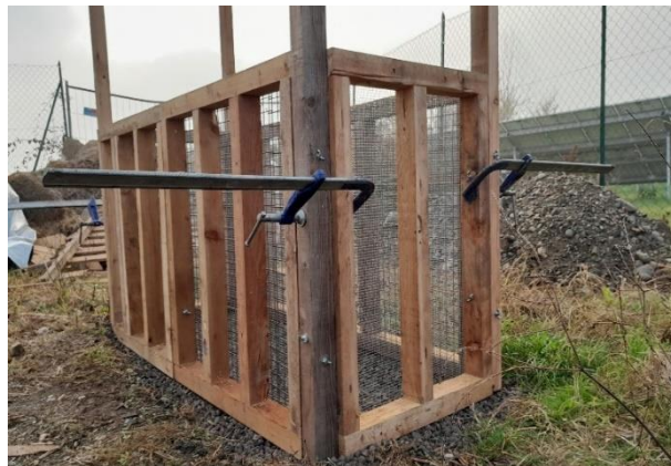
Figure 70 : First floor of formworks fixed with the wooden corners
