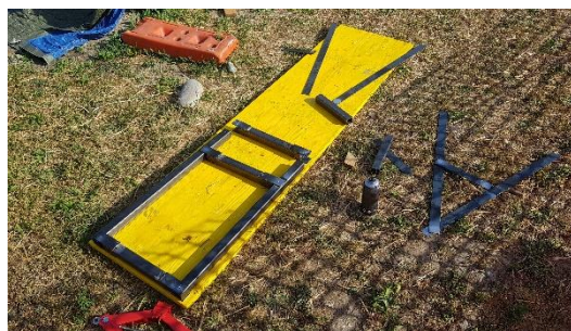
Figure 26 : Self construction of the press
