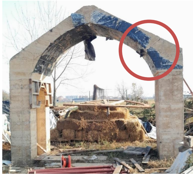
Figure 96 : West elevation of the arch
