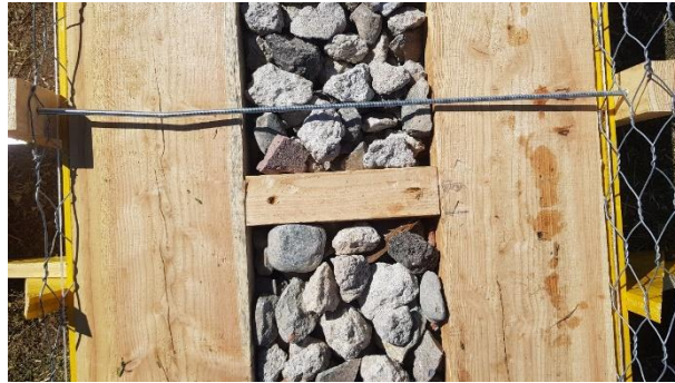
Figure 143 : Spacing of the beams
