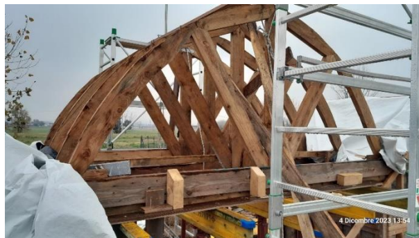
Figure 80 : Fixing centrings by cross bracings
