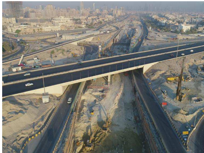
Fig. 4. The monitored concrete highway bridge.
