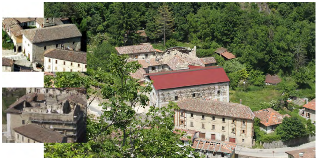
Fig. 1. San Francesco Church before and after the 2016 earthquake.
