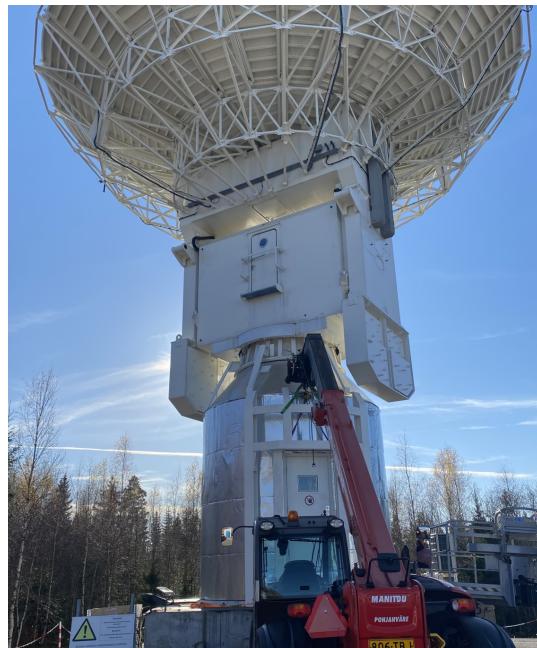
Fig. 2 Work on the telescope pedestal insulation (October 2022).
