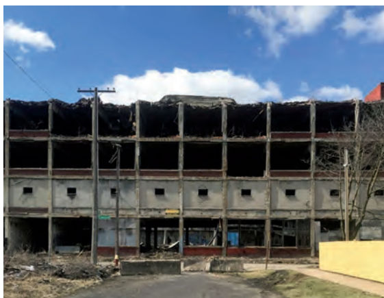
Fig. 9 Ex stabilimento Packard, Detroit, stato attuale, 1903-2019. Former Packard plant, Detroit, current status, 1903-2019. (© Gian Luca Meli, 2019)
