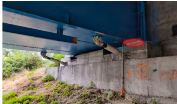
Fig. 4. Unidirectional longitudinal bearing at abutment 1.
