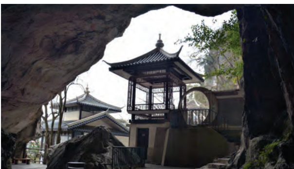
Figure 8. The Qixia Pavilion in Seven Stars Scenic Area. Produced by the author.
