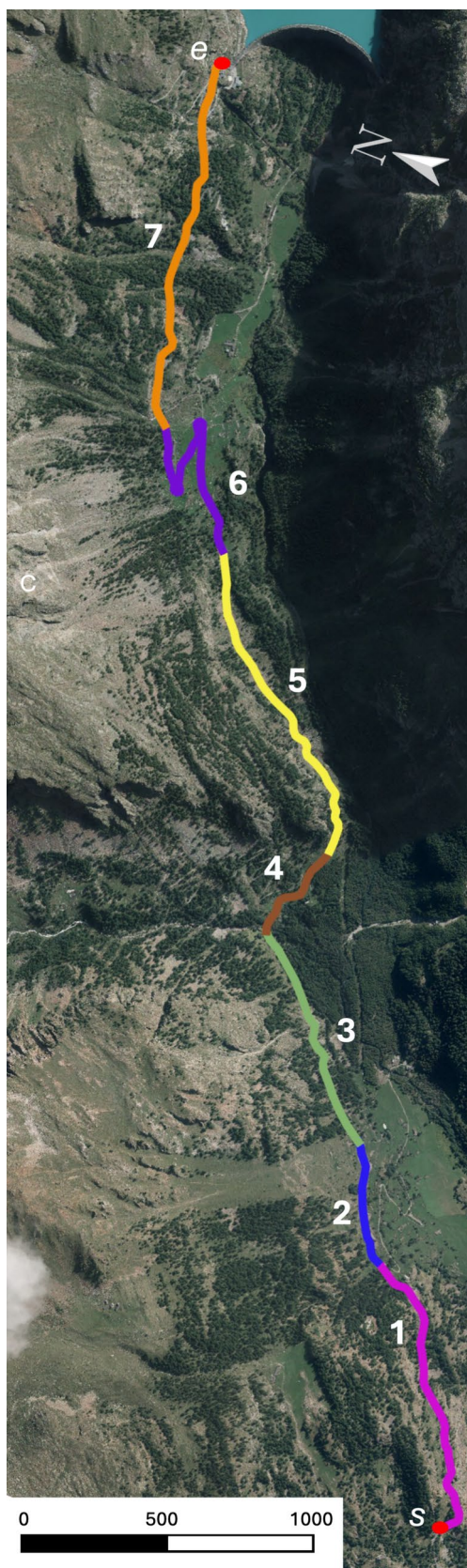
Fig. 5 Aerial view of the valley and indication of the seven different road sections. Points s and e are marked. The letter C indicates the top slopes of Becca di Châtelet
