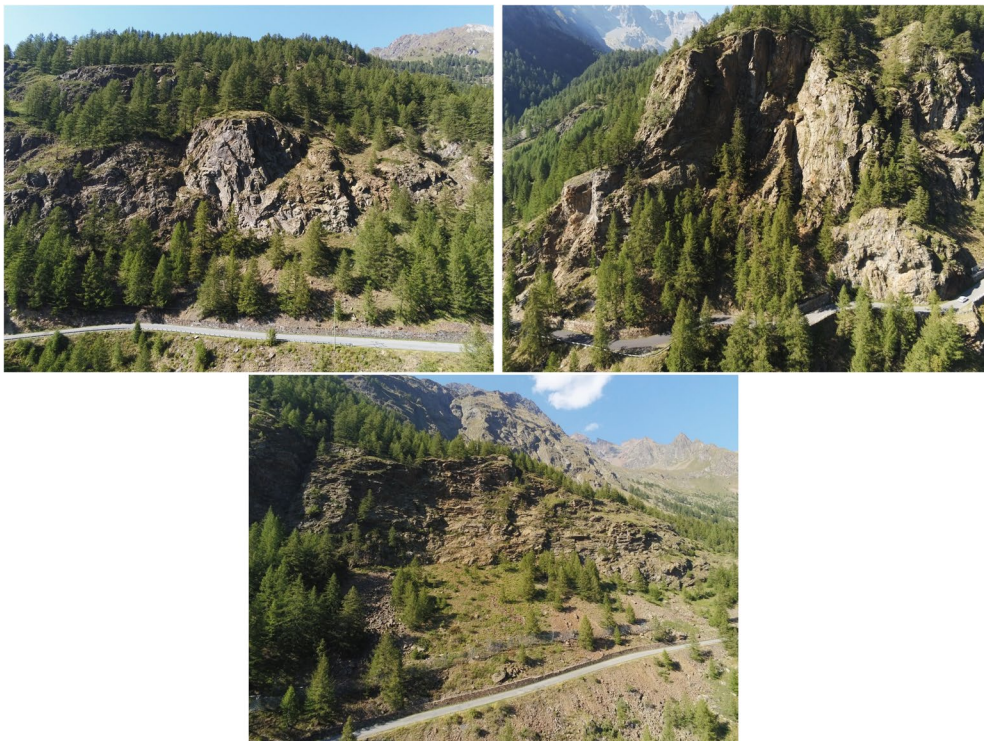
Fig. 4 Three aerial views of the road and the upslope cliffs
