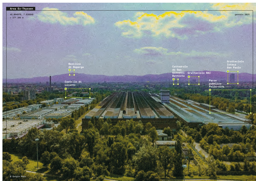
Fig. 1. Area capture of the site, framed in relation to the defining elements of the city of Turin. Source: Google maps (elaboration by the authors).
