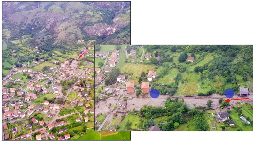
Fig. 9 Photographs documenting the debris-flow event of June 2018: the images show the flooded area and the affected buildings. The red arrow indicates the flow direction, while the blue circles mark the locations of destroyed structures
