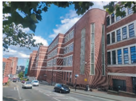
Figure 2. Broad Lane Building (Harpin).
