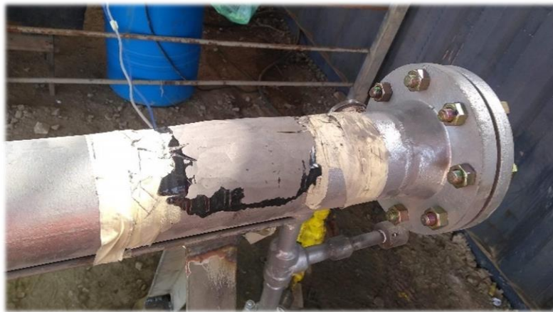
Fig. 3. Repaired region after the patch cure.
