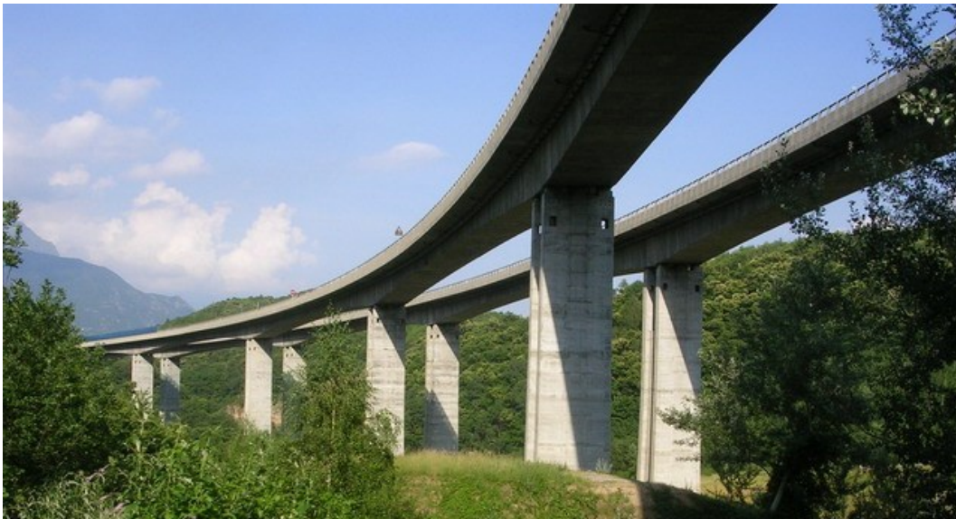
Figure 6-24: Picture of the viaduct.
