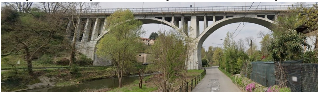
Figure 6-10: Picture of the bridge.
