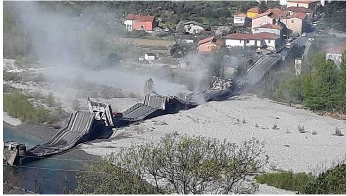
Figure 1-5: Collapse of the Capriogliola bridge.
