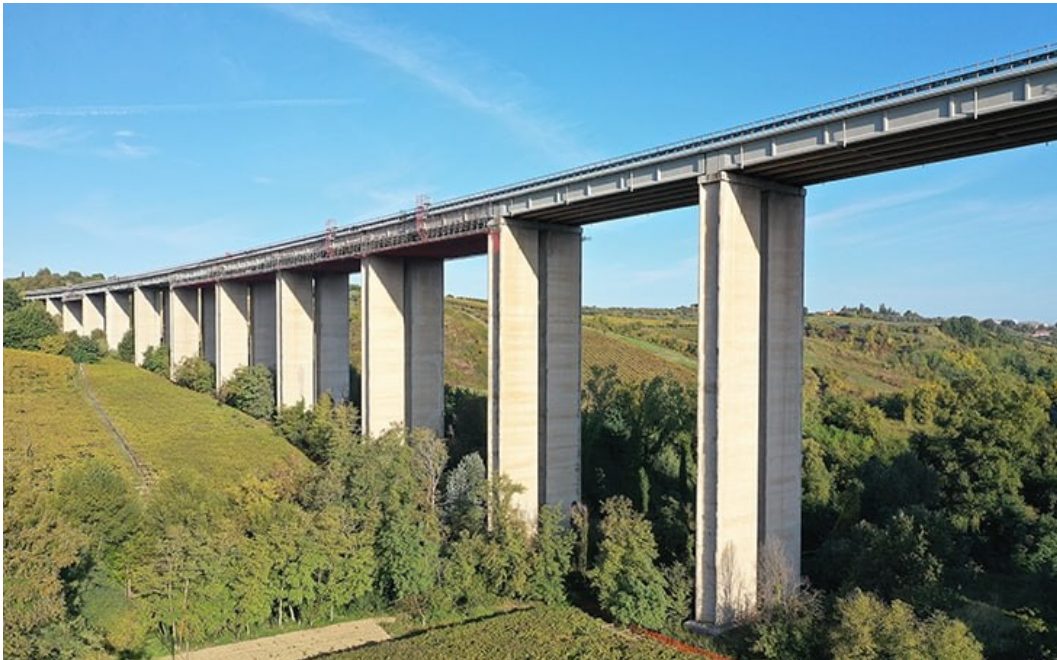
Figure 5-1: Picture of the viaduct.
