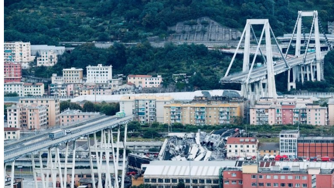
Figure 1-4: Collapse of the Polcevera bridge.
