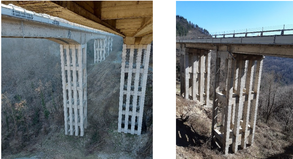
Figure 4-1: Pictures of the viaduct.
