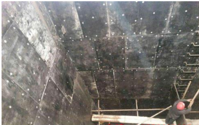
Fig. 2. Inside of coal bunker
