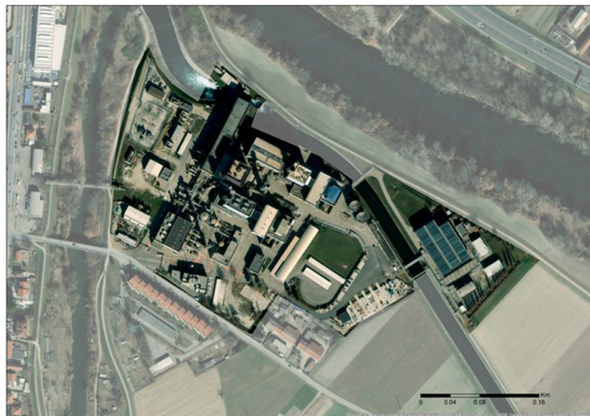
Fig. 9. Satellite view of the critical energy infrastructure used as a case study. Source: modified from [61].
