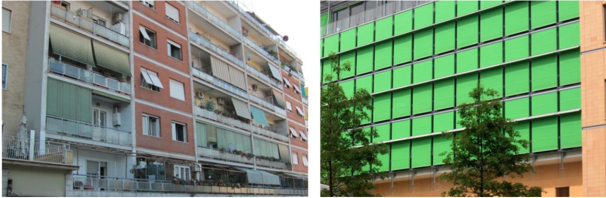
Figure 2: Individual low-cost external blinds in a social housing building in Rome, Italy (left) and the fully automated shading façade at a newspaper headquarter in Milan, Italy (right) [1].
