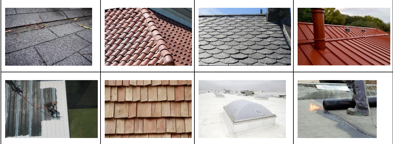
Figure 3: Examples of common roofing products (top row, left to right: fiberglass asphalt shingle [23], clay tile [24], slate[25], standing-seam metal bottom row, left to right: field-applied coating [26], wood shake, single-ply membrane [27], asphaltic membrane [28]).
