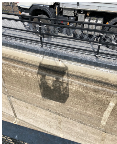
Figure 2. A crane with a gondola was used to reach all parts of the dam to place the markings.
