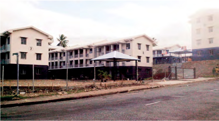
The roof of the buildings, as well as the windows, are equipped with overhangs for rain protection.
