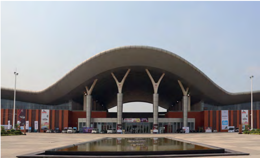
The façade made of red terracotta tiles is protected by a suspended big roof.
