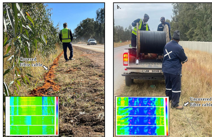
Figure 3—Deployment of distributed acoustic sensing (DAS) fibre optic cable along the nodal system profiles. (a) Insert shows the recorded signal from the covered fibre optic cable with soil and the signal is less noisy (b) Shows the uncovered fibre optic cable
