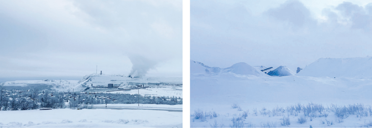
Fig. 5: Caving deformations (left) Dumping of tailing piles (right)
