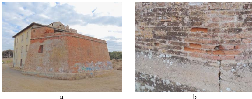
Figure 5 – Forte di Marina di Castagneto (a); particular of biological growth phenomena (lichens) and brick erosion (b).
