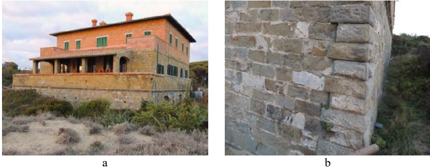
Figure 3 – Forte delle Marze (a); detail of the Pietra Serena ashlars of the bastion scarp wall (b).
