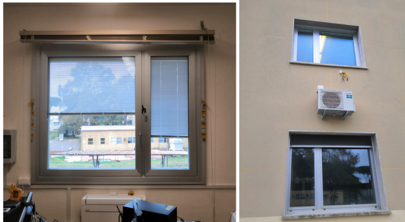
Fig. 3. Inside view of a W2 window with the solar shading device partially activated (left) and outside close-up of the facade, where the intrados of the windows are clearly visible.
