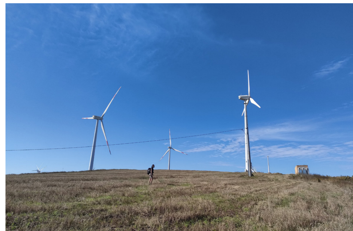
Fig. 3. Extensive wind farm installation, 2022, Avigliano, Basilicata; image elaborated by the author.
