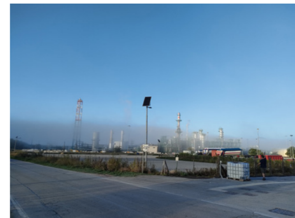
Fig. 2. Val D'Agri Oil Centre (COVA) noise and unbearable air condition, 2022, Viggiano, Basilicata; image by the author.
