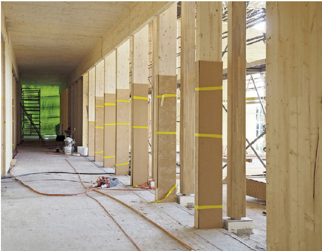
Fig. 3 | Construction site photograph of the central distribution corridor, showcasing the doubling of the vertical structure next to the double-height outdoor terrace (credit: Blumer Lehmann | Claude Hausammann, 2017).
