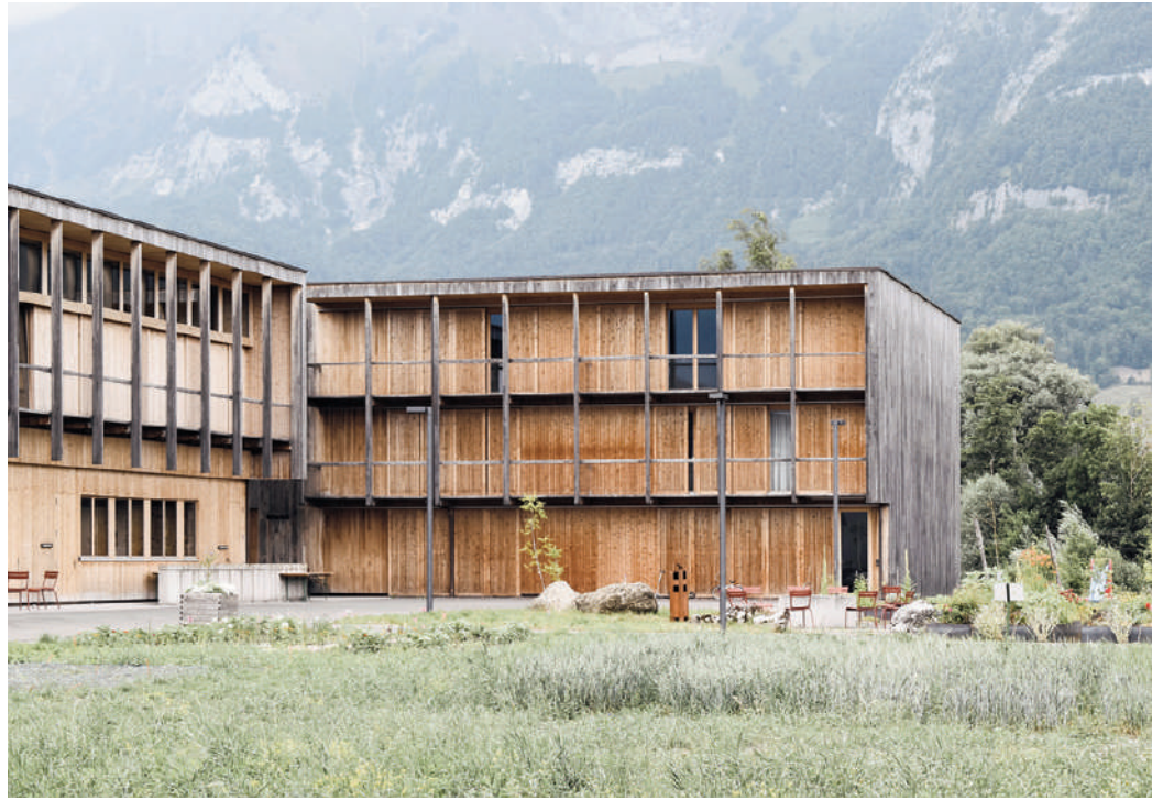
Fig. 2 | The Landwirtschaftliches Centre St. Gallen viewed from the inner courtyard. The image depicts the connection between the two-storey teaching wing and the three-storey dormitory wing (credit: the Authors, 2023).
