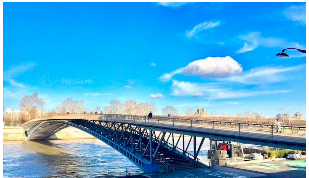
Figure 2. Solférino Bridge in Paris (FR) looking north.
