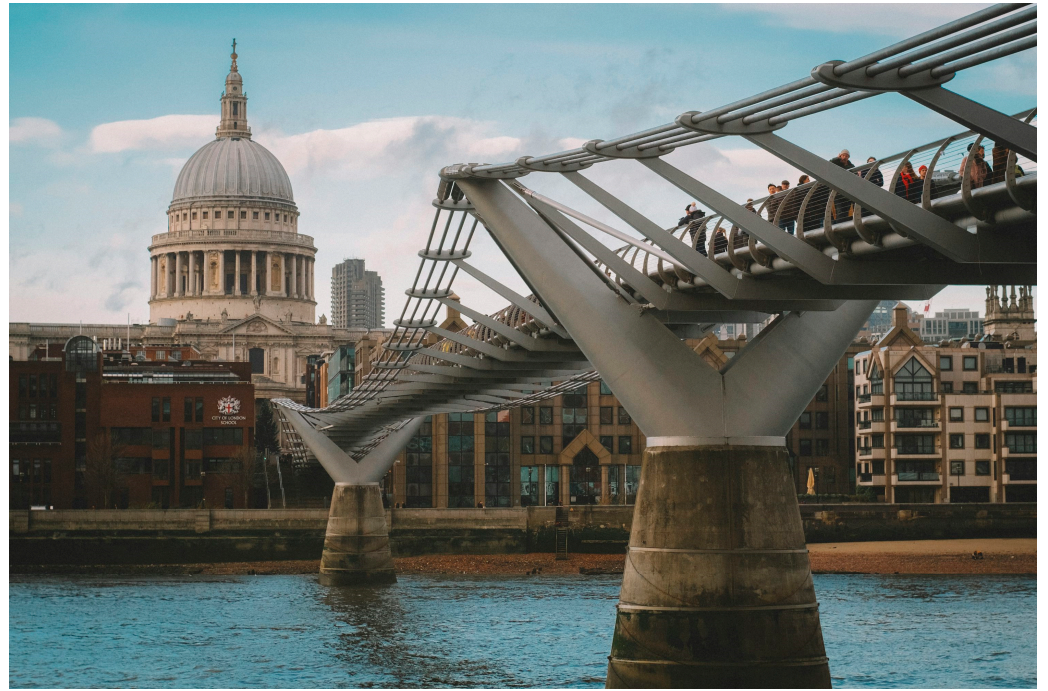
Figure 1. Millennium Bridge in London (UK) looking north.
