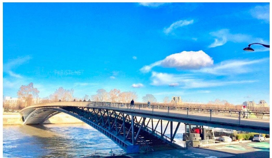
Figure 2. Solférino Bridge in Paris (FR) looking north.
