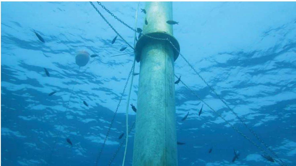
261 Figure 6 - Catenary mooring system of the model, including delta connections [29]
