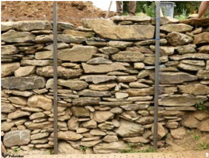
9. Construction of a dry stone wall during a workshop dedicated to the topic. Gaëlle Carvalho/Palombar 2019.
