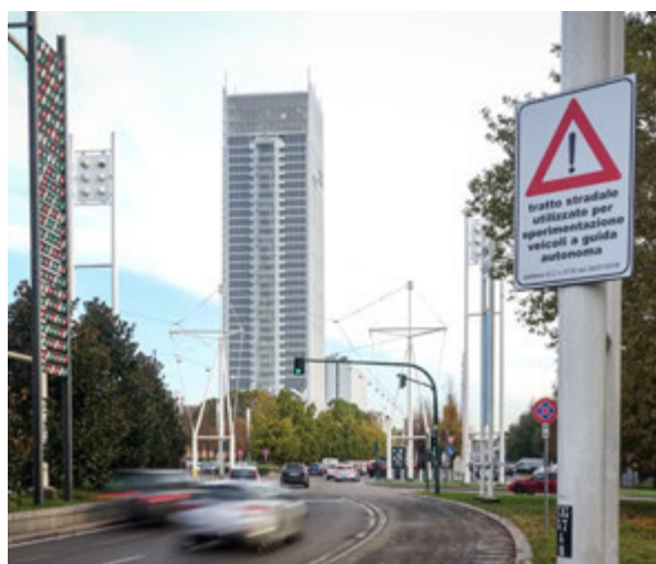
Figure 1. A road in Turin equipped with technologies needed to test autonomous vehicles (Source: Scudellari et al., 2020).
