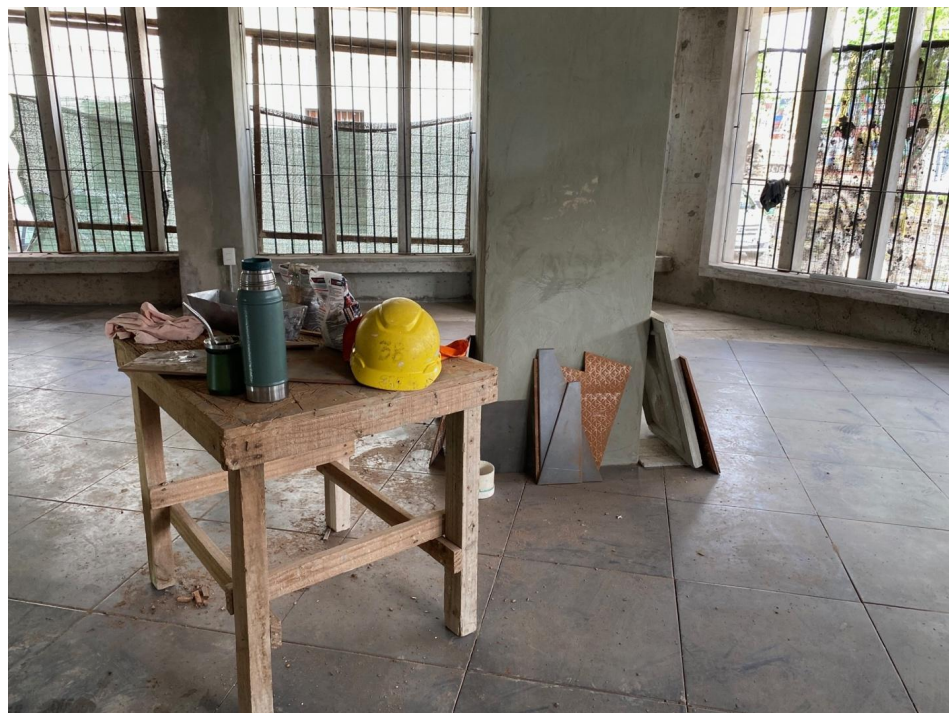
Visit UFAMA CORDON 1 cooperative mutual aid construction site. Photo: Ana Vilenica
