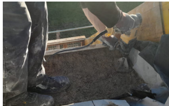
Figure 5. Homemade electric tamper.
