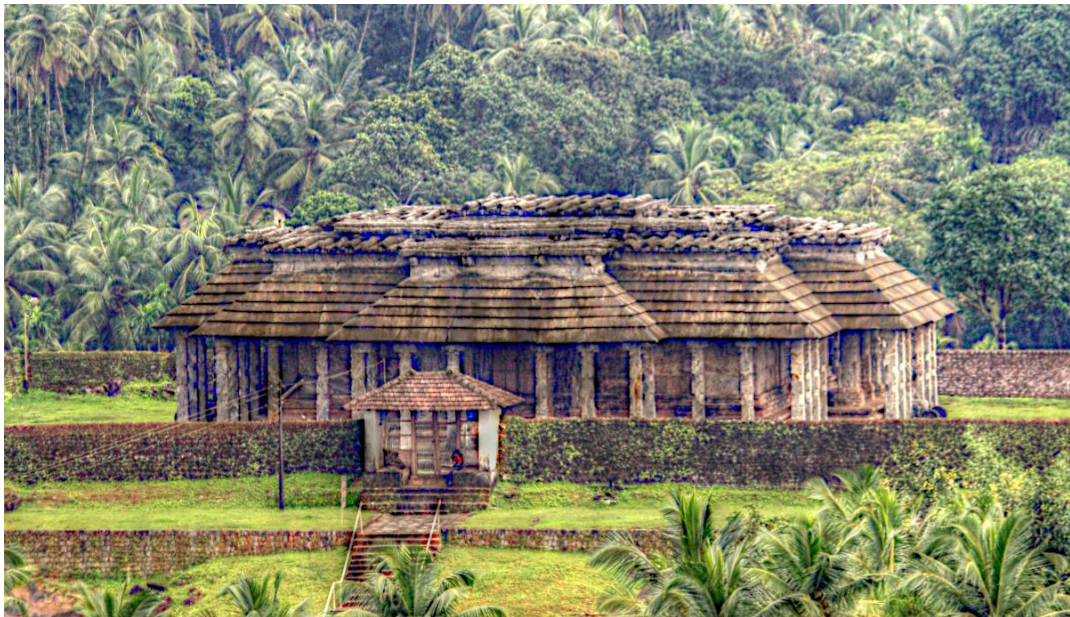
Fig. 11. Chaturmukha Basadi is built in a form of a square mandapa or hall and has 4 identical doorways with a lofty doorway and pillared entrance on each of its four sides. There are a total of 108 pillars inside and outside the temple. Photograph courtesy Anooprata maker, CC BY-SA 3.0 ( link to the photograph )
