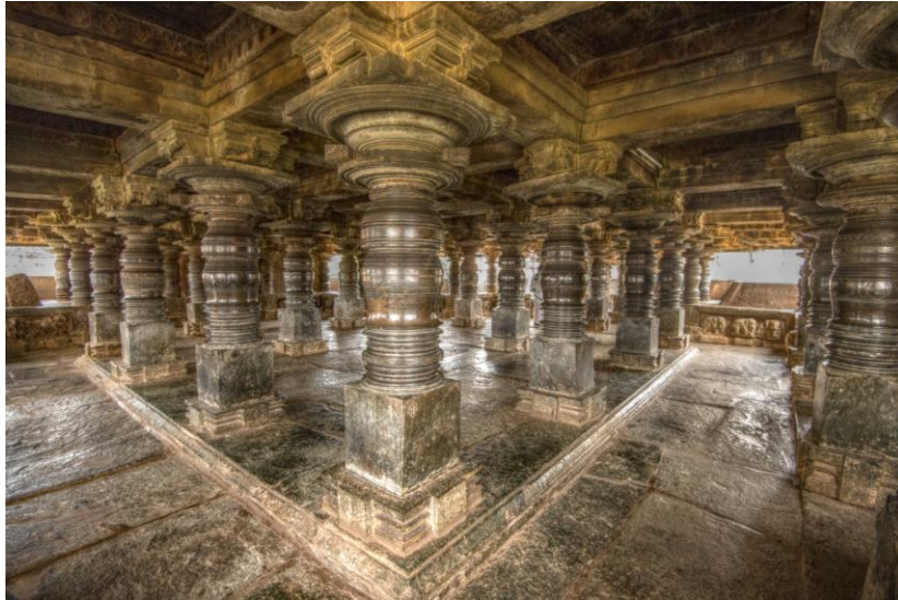
Fig. 11: The Veera Narayana Temple and the turned pillars “in the ranga-mantapa between the Venugopala and Yoga Narasimha shrines”, as explained by Bikashrd who kindly provided the photograph under CC BY-SA 4.0 License ( link to the phptograph ). Pillars are 108 ( Video )
