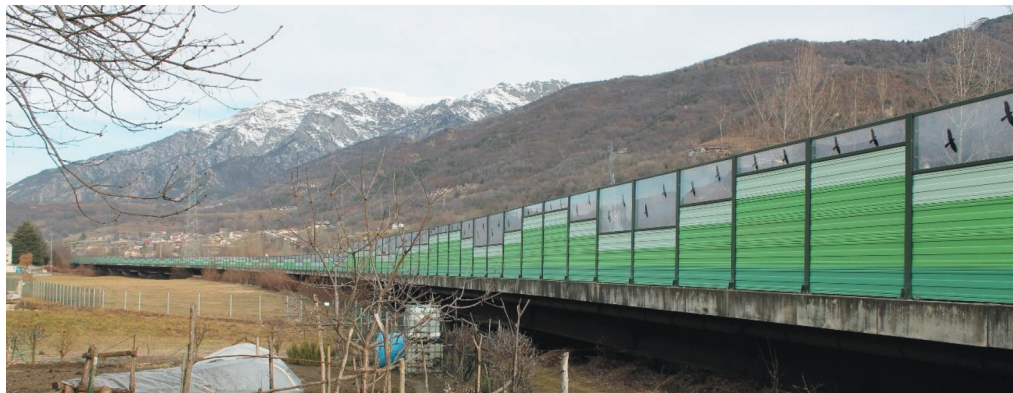
Figure 1. Side view of the Inverso Pinasca bridge in its full length, as captured during preliminary in situ surveys (February 3 rd , 2023).
